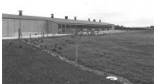
Free range showing electric fence.
